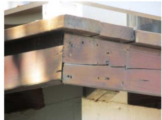
Wood balcony deterioration, cracks and deck board deflection
