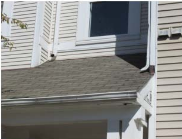
Downspouts draining onto lower elevation roof
