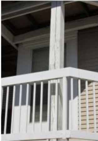
Wood post cracks and deterioration
