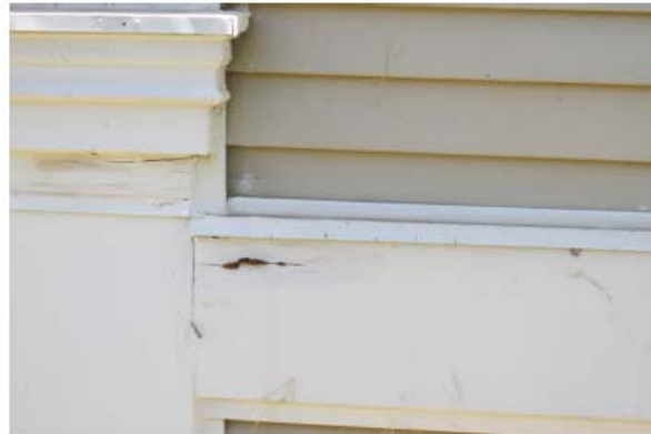
Trim deterioration
