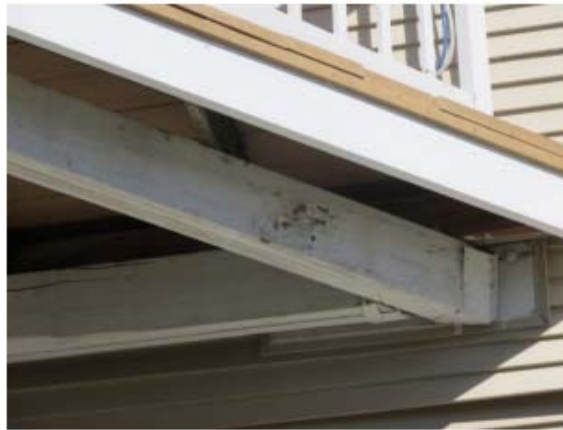
Wood frame deterioration
